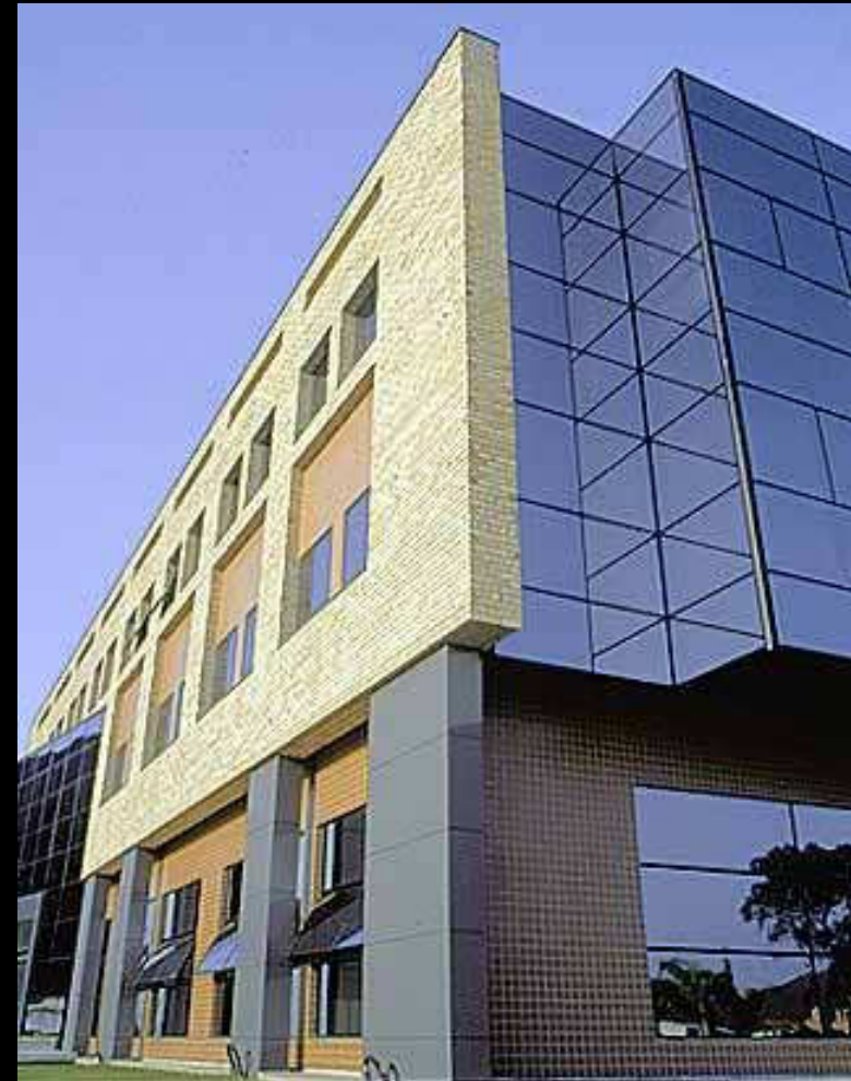
79 – Portobello Office Park
