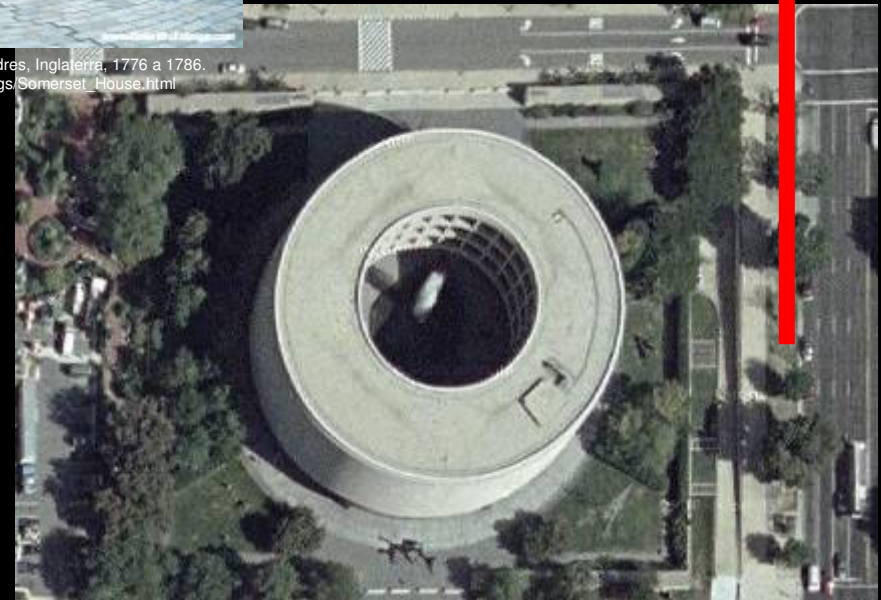
Museu Hirshhorn, de Gordon Bunshaft/ SOM, em Washington, D.C. 1974 Fonte: http://www.greatbuildings.com/buildings/Hirshhorn_Museum.html
