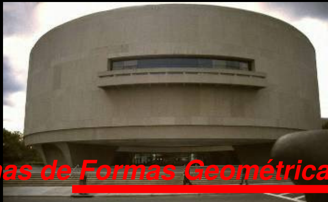
Museu Hirshhorn, de Gordon Bunshaft/ SOM, em Washington, D.C., 1974. Fonte: http://www.greatbuildings.com/buildings/Hirshhorn_Museum.html
