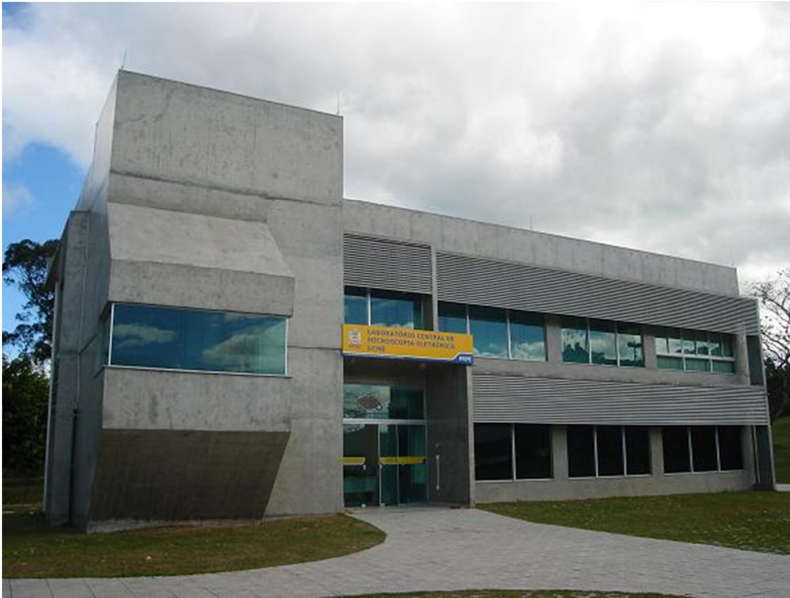
Figura 04: Fachada Principal LCME (Norte)
